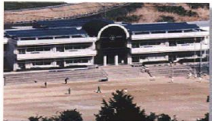
Solar cell capacity: 30 kW
