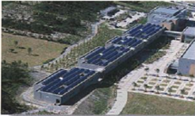
Solar cell capacity: 250 kW
