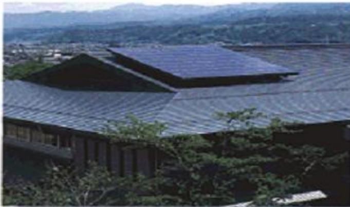
Solar cell capacity: 10 kW
