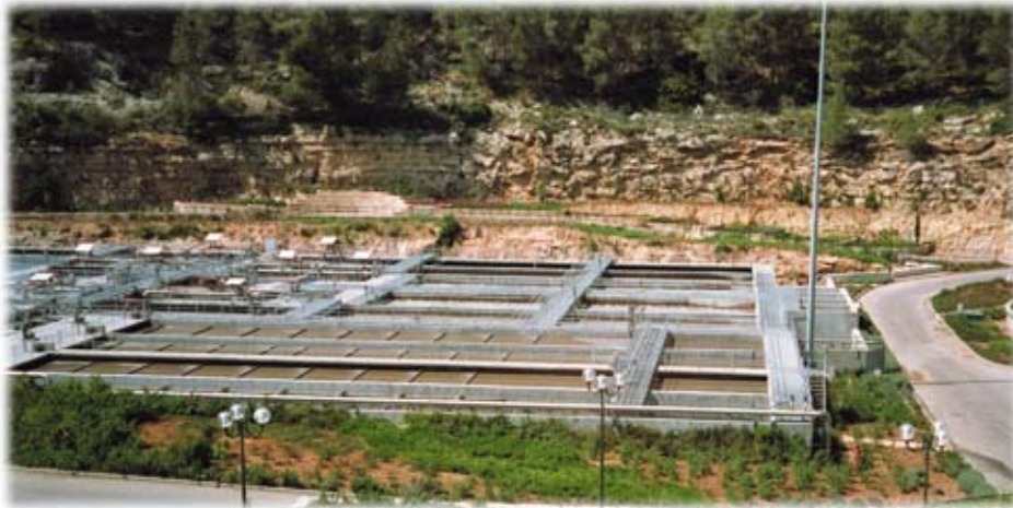
Wastewater treatment plant
